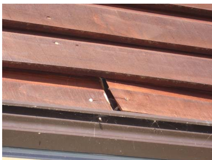
Warping of band sawn plain sawn Radiata Pine
